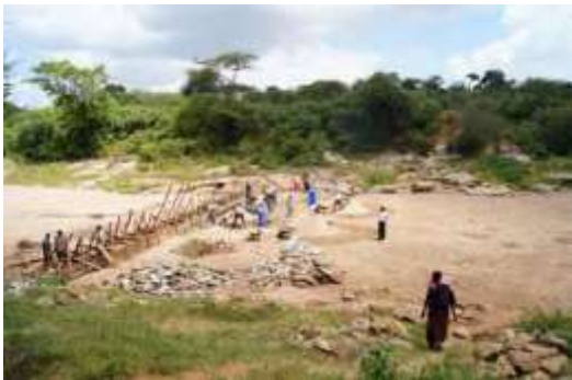
Sanddamm in Bau
